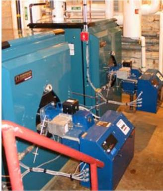
Even at start-up a big difference could be noticed – the boiler room temperature had dropped 30-degrees from the previous boilers. The MPC's 4-inch insulation blanket insulates the boilers so well that the jackets stay cool to the touch, and the boiler room at the Hershey Mansion is now a much more comfortable place to work.
