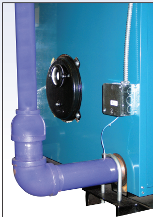
Return Sensor Monitors Boiler Return Water Temperature
