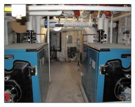
efficiency model MPC9 boilers (up to **88.6% efficiency**). The old boiler operated at minimal efficiency, especially during the spring and fall when the building demand only required partial load. The mansion, built during the dawn of electricity, used a gravity feed system with large 18-inch supply and return mains. These large supply and return mains divide up into a network of several
