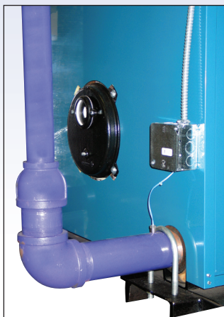
Return Sensor Monitors Boiler Return Water Temperature
